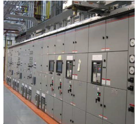
Automatic Paralleling/Loadsharing Switchgear
